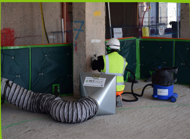
HEPA Filtration can help protect against silica & wood dust.
