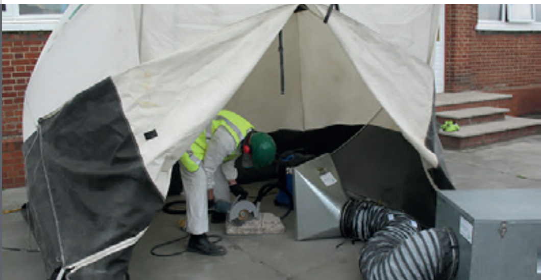
A negative pressure system using a dust containment enclosure.
